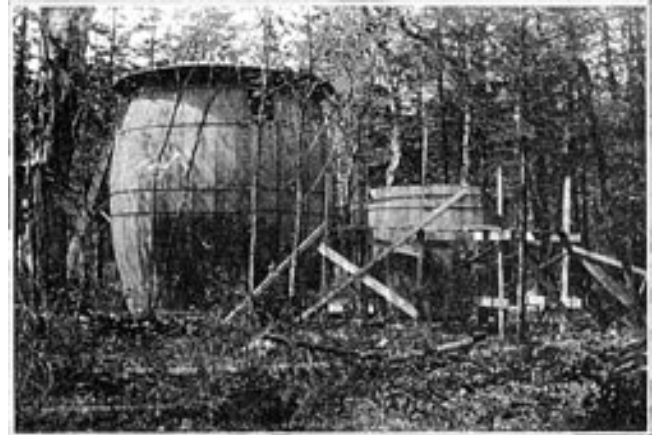
"Then they began cutting windows and doors—and things commenced to happen."
